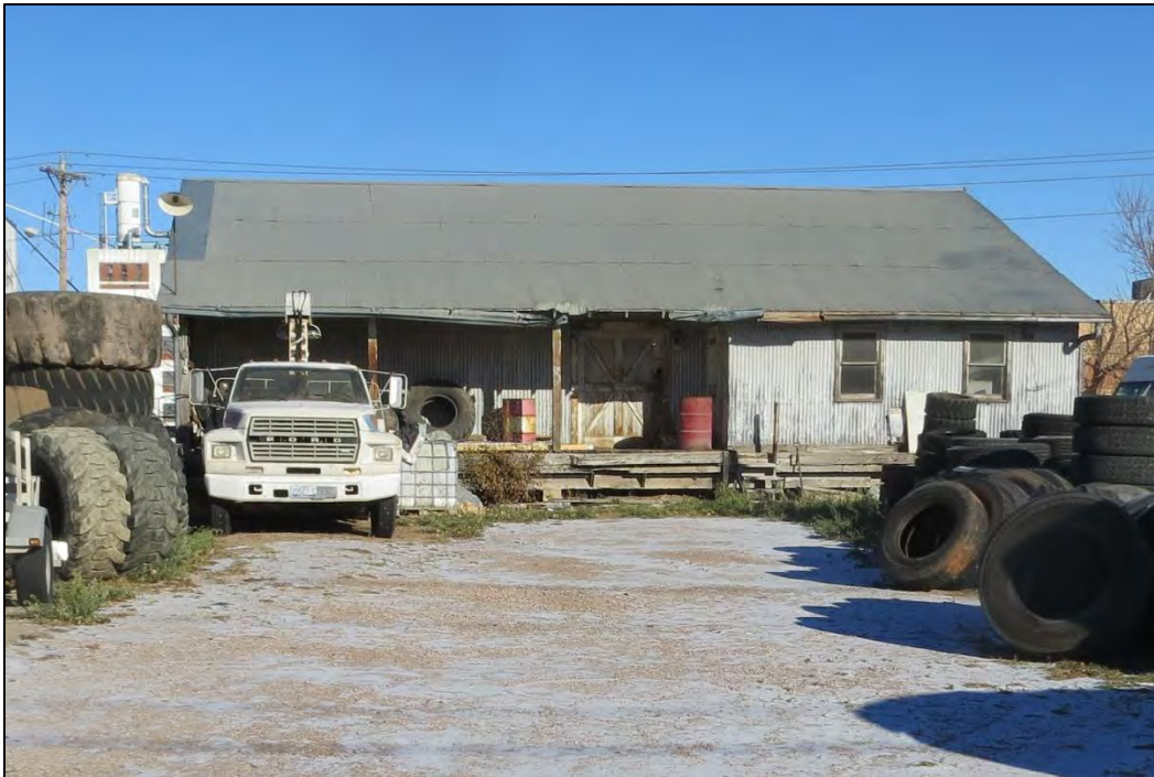
Figure 39. 415 4 th St. facing northeast. M. Carpenter 12/4/2016.
