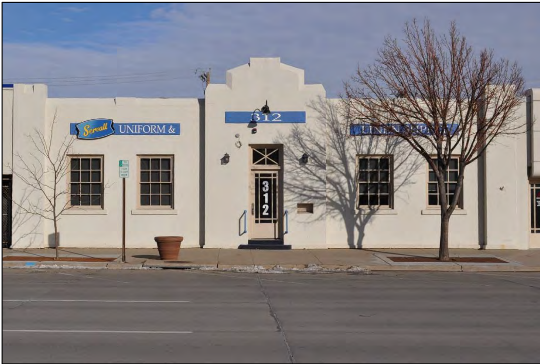
Figure 27. Site 18711 Structure 23506 at 312 Main Street, also known as the Rapid City Laundry or Kellogg Laundry, was listed on the National Register in 1995. This Art Deco structure retains its historic character.
