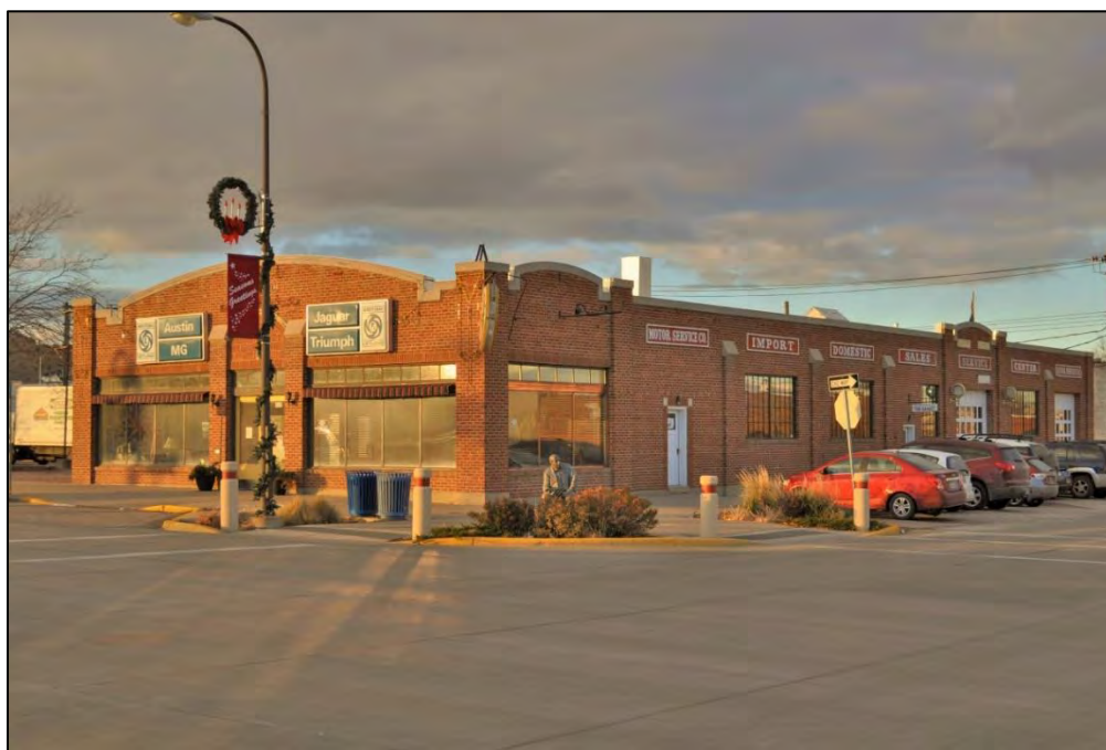
Figure 29. The Motor Services Company building at 402 St. Joseph looking northwest. B. Moloney 12/14/2016.
