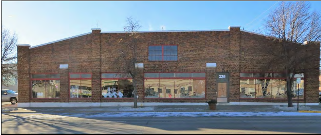
Figure 34. 329 Main St. facing south. M. Carpenter 12/13/2016.
