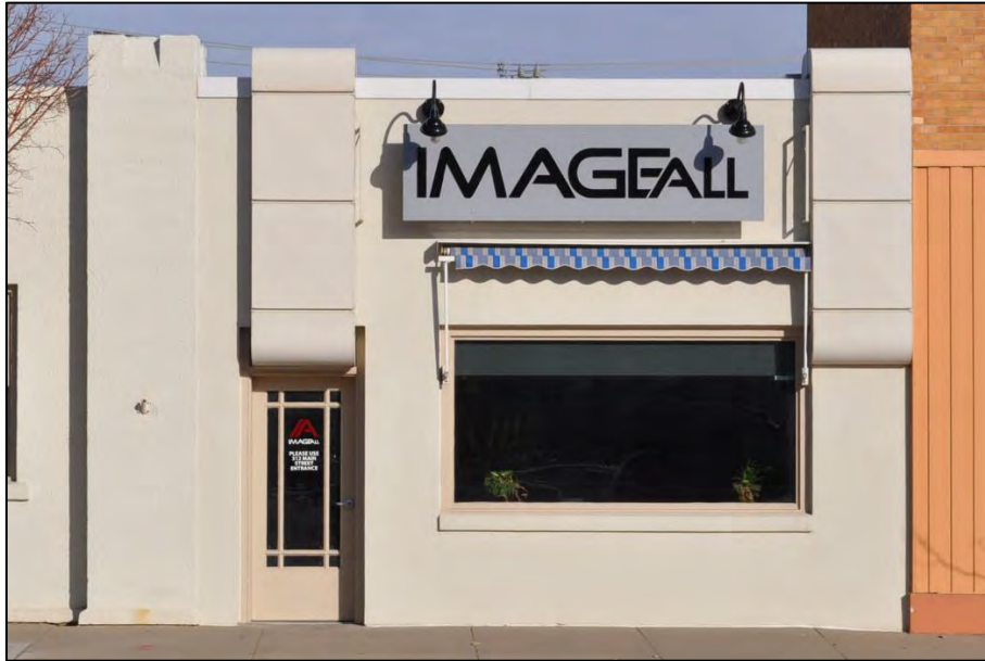
Figure 28. The 1945 east addition to the Laundry was also designed by architect James Ewing. B. Moloney 12/02/2016.
