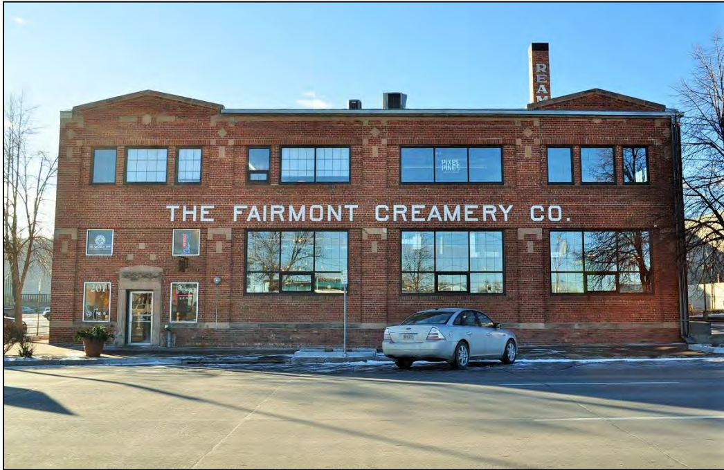
Figure 32. Site 28755 Structure 32306, 201 Main St. facing south. B. Moloney 12/14/2016.
