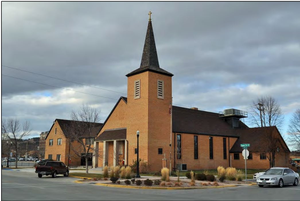
Figure 41. Trinity Lutheran Church at 402 Kansas City Street facing northwest. B. Moloney 12/02/2016.
