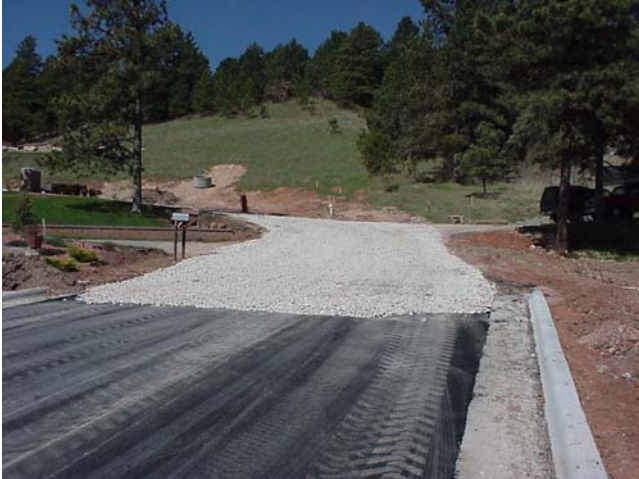
Construction entrances prevent trackout
