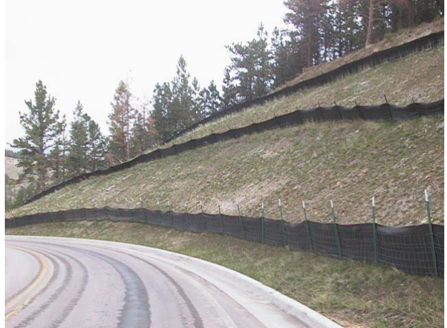
Silt fences hold soil on the site
