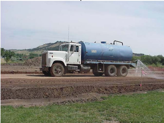
Use water to control dust
