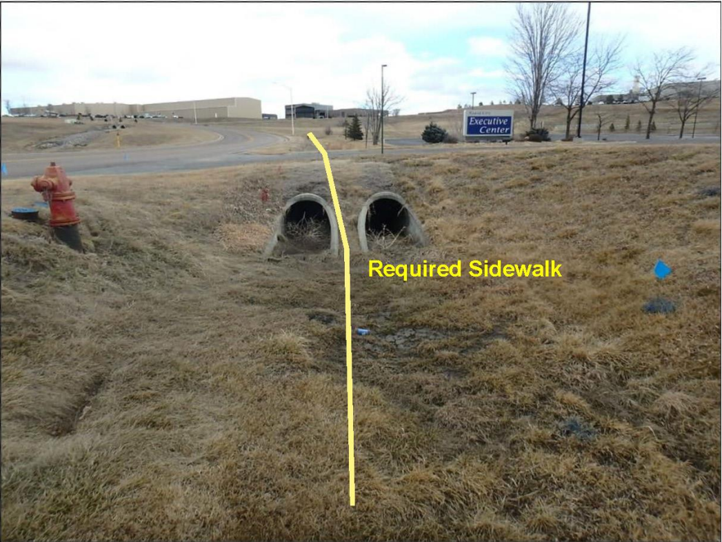
Figure 4: Drainage ditch on Concourse Drive looking North
