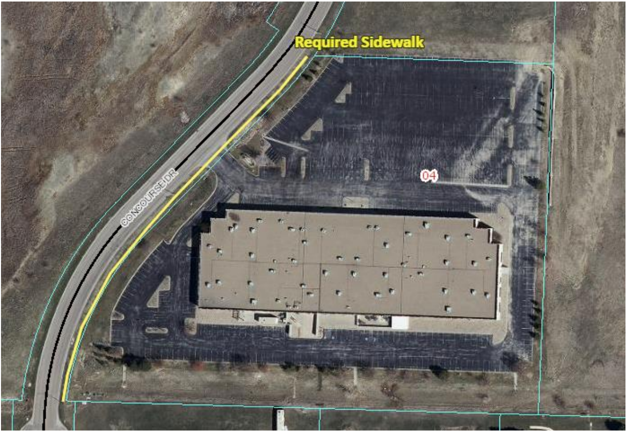
Figure 2: Approximate Location of Sidewalk
