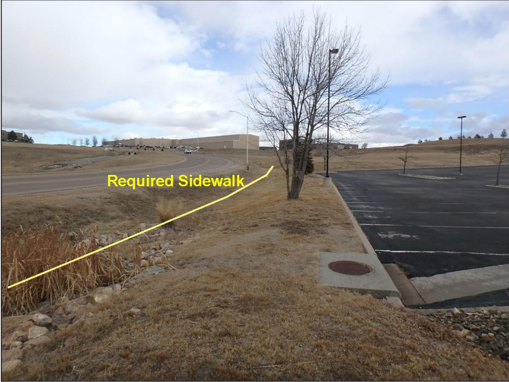
Figure 3: Drainage ditch on Concourse Drive looking North
