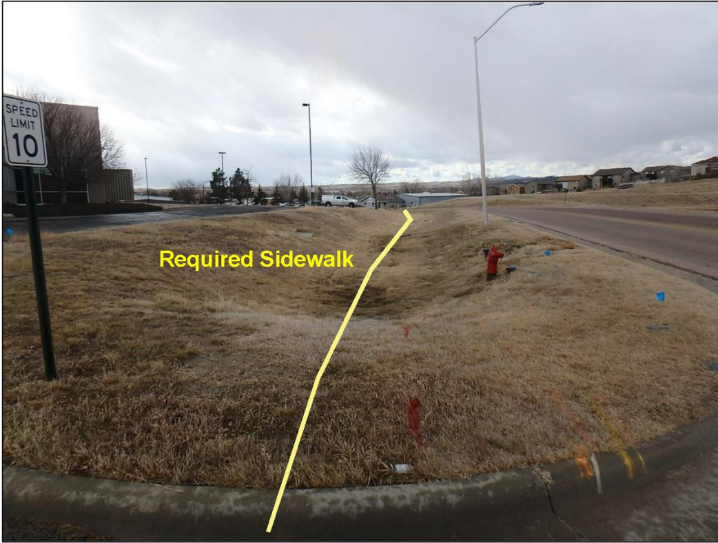
Figure 5: Drainage ditch on Concourse Drive looking South
