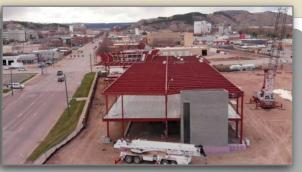
The Ascent Innovation Center is under construction on Main Street and East Blvd. The new business incubator will have 48,595 sq. ft. on two floor. Steel continues to be placed, with structure stability being a major effort. Completion is anticipated in fall 2020.
