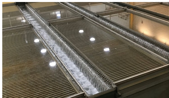
Sedimentation Basin at the Jackson Springs WTP. This is one step in the conventional water treatment process.
