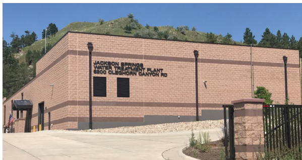
Jackson Springs Water Treatment Plant
