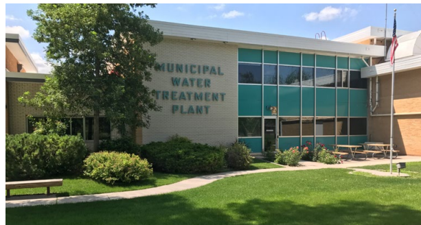
Mountain View Water Treatment Plant
